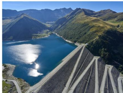
Grand'maison Source: encyclopedie-energie
